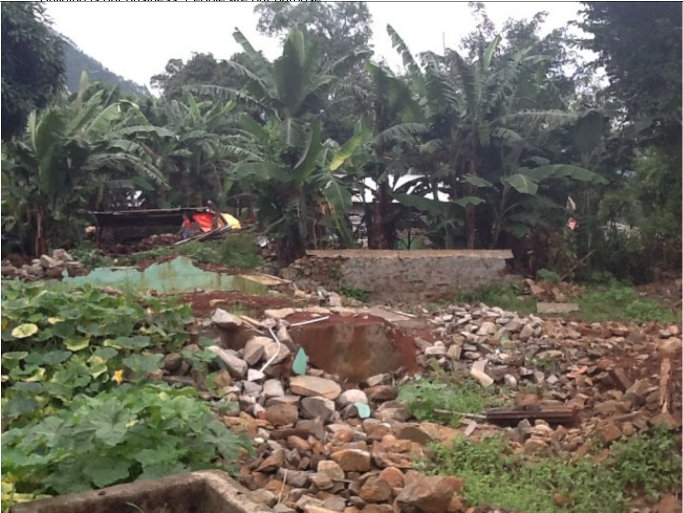
A village home in Gurkatar, turned to rubble by the quake.
